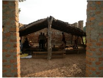
Existing facility inside the walls of new building
