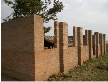
New sanctuary under construction
