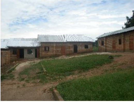
Original building to the right with the three rooms finished so far in 2014 in the back
