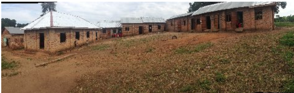
Panoramic view today. Church building is the extreme left. The style of roof on the original school building and the new ones has been changed to handle the extreme wind loads in this part of Uganda. We are seeking to raise funds for the next round of building which we plan to be in December. It will provide more housing for faculty and finish the doors and windows in all the existing buildings
