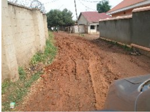
Roadway to church
