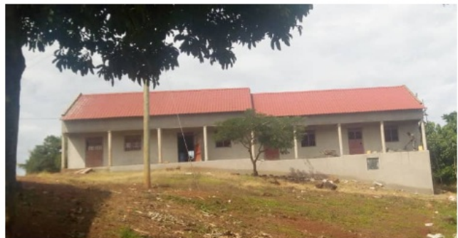
Building now finished except for painting
