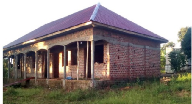
Current stage, needs windows and doors and plaster and painting
