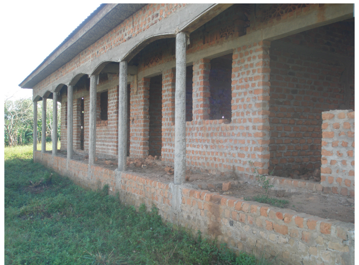
The newest school building progress
