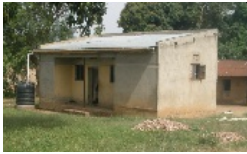
Finished project as seen from road
