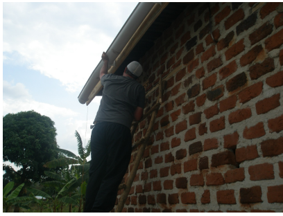
Fred working on a gutter project
