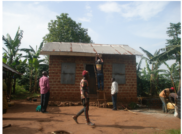
Another of the rain tank projects in progress
